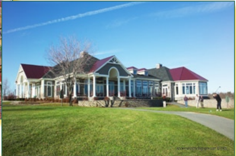
Van Patten Golf Clubhouse Construction Management
